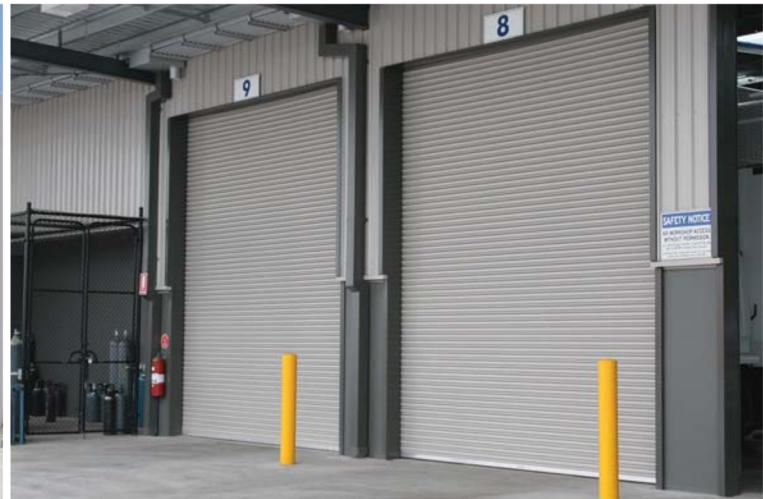
Series 75 Roller Shutters consist of individual interlocking steel slats, providing high strength security for commercial and industrial applications such as factories, loading docks, workshops and warehouses.
